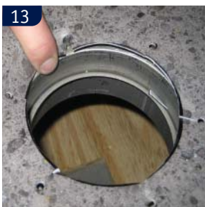
13 Pres vinylen ned Bend the vinyl into the drain
