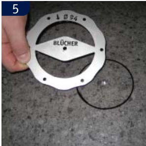
5 Optegn hullet (ø94 mm). Mark up the center hole to be cut.
