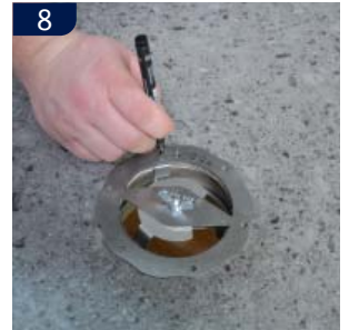
8 Marker hullerne Mark up the holes to be cut.
